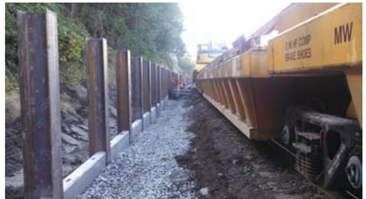
BNSF is building a wall to hold back a slide-prone hillside at milepost 29.5 between Everett and Edmonds.
